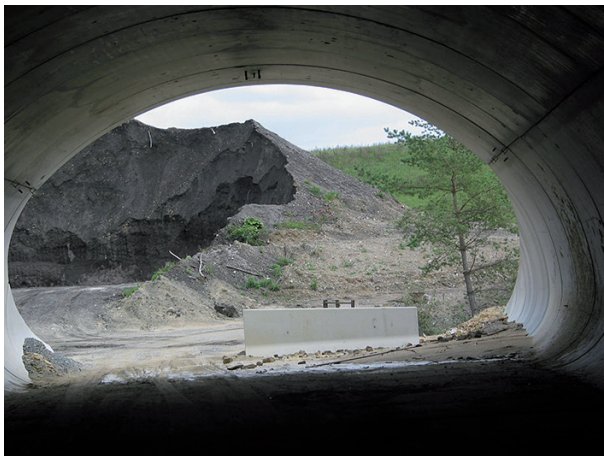
Fig. 3. The Sulkov landfill residue viewed from new motorway in 2002. Photo Jan Kopp.
